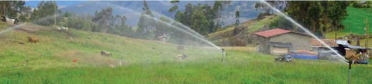
Technified Irrigation System - Barrojo Community
